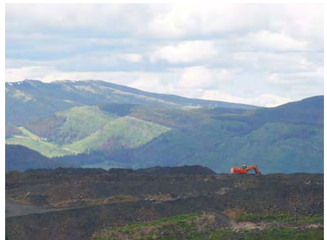
Figure 2.12. Site Preparation at Willow Creek North Zone.
