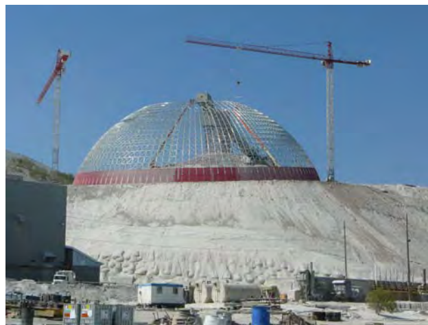
Figure 4.5. Geodesic domes over ore stockpiles being installed at the Highland Valley Copper mine near Logan Lake.
