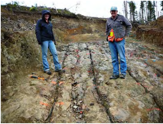
Figure 4.20. Consultant Grant Crooker showing the sawn channel samples in the Bonanza Trench at GoldCliff Resource Corp's Panorama Ridge property near Hedley.
