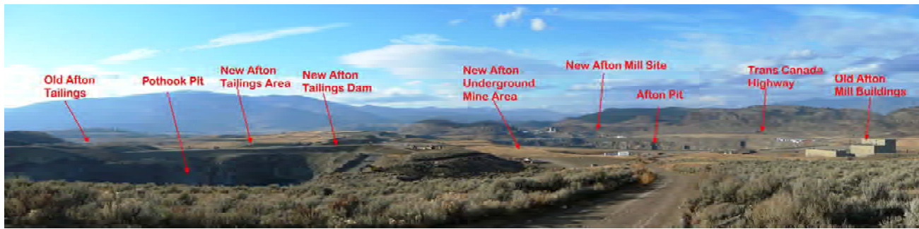
Figure 4.6. Panorama of the New Afton mine development of New Gold Inc just outside Kamloops showing major areas of work.
