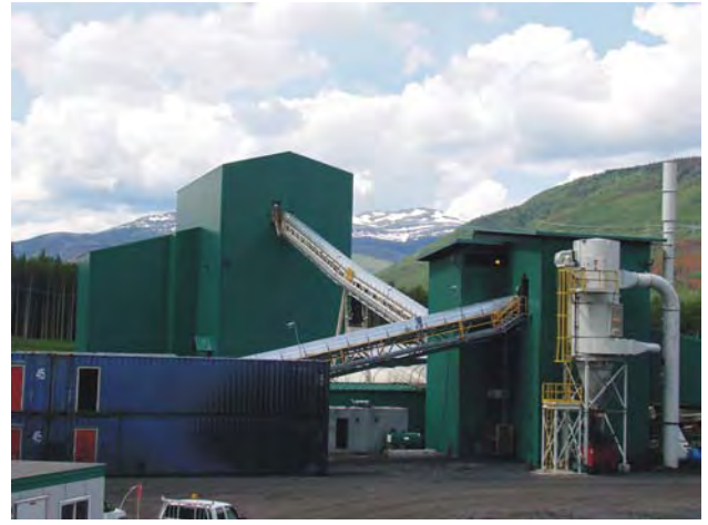
Figure 2.8. Grizzly, crusher and wash building at the Willow Creek mine site.
