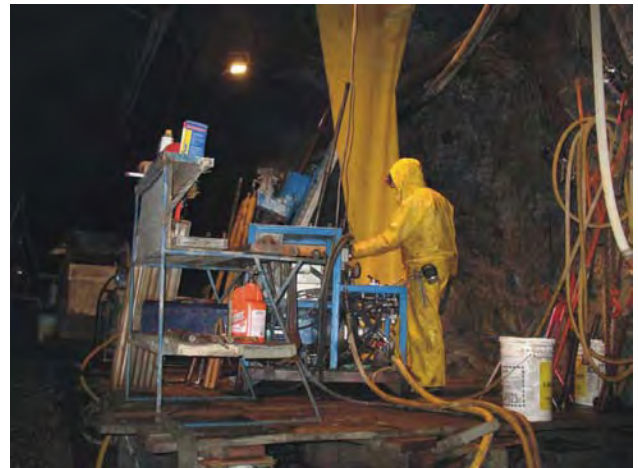
Figure 5.10. Drilling underground at Myra Falls. Exploration focused on targets close to existing mine infrastructure in the latter half of 2008.
